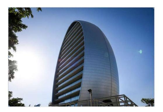
At its final level of development, the model provided the basis for the panelisation and the panels fabrication and the coordination of the whole cladding build-up system.
